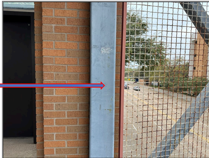
2. View of Support column on South Bridge, SE.
